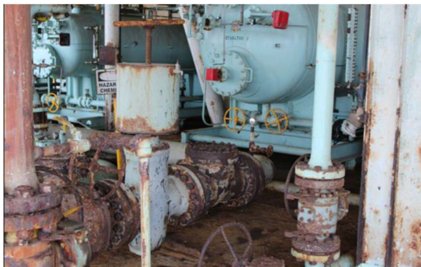
Figure 5—Corrosion on Platform Hogan (GAO, 2024)
