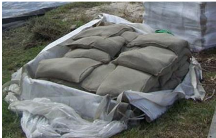
Figure 2. 3:1 Sand-to-Cement Burlap Bags
