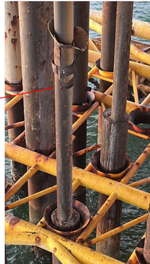
13-3/8 Conductor Failure point
