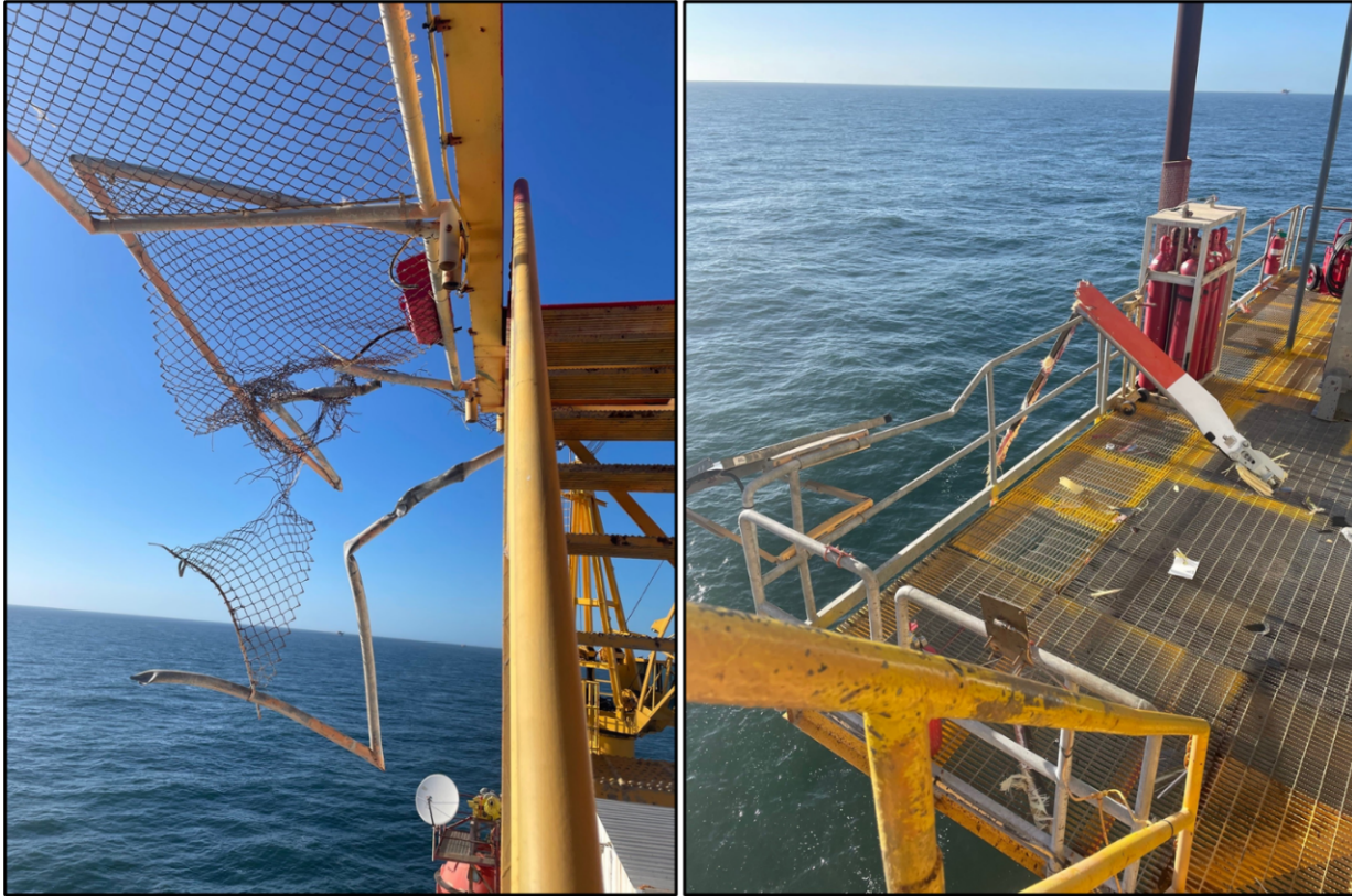
Image 2a (left) – Damaged chain link perimeter skirt on southwest corner of helipad Image 2b (right) – Portion of a main rotor blade found on the deck below the helipad
