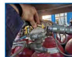
Incident 2: Failed Hose Connection on Bottle Rack.
