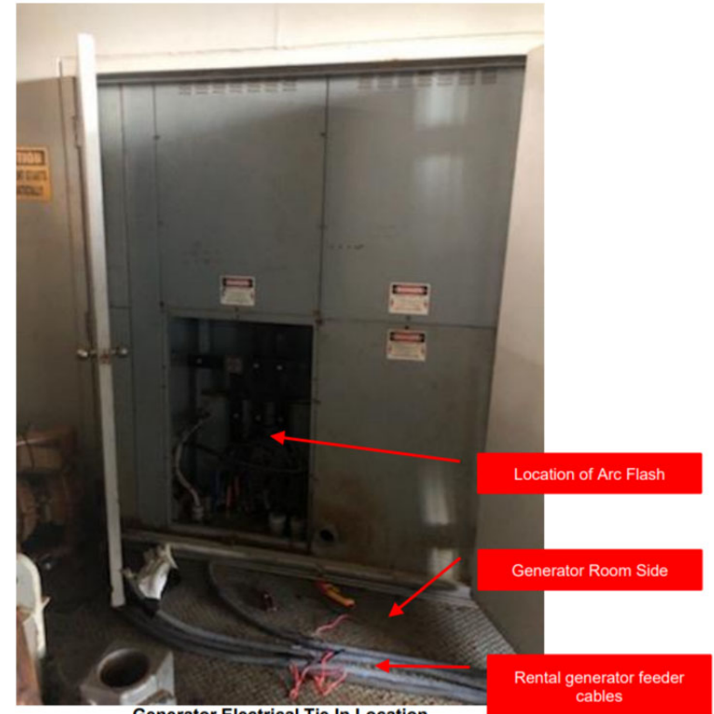
Generator Electrical Tie In Location
